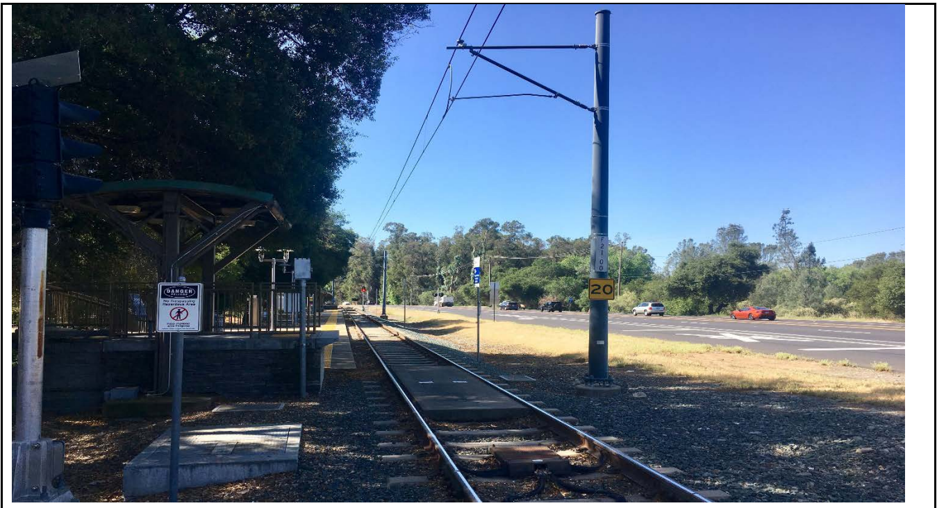
Viewpoint 4. Looking south at the Glenn Station. Trees, shade structures, and the concrete boarding platform, along with the light rail tracks and the OCS, and the proposed location of the new boarding platform, are visible in the foreground and middleground. Folsom Boulevard and trees in the Folsom Lake SRA are visible in the foreground, middleground, and background.
