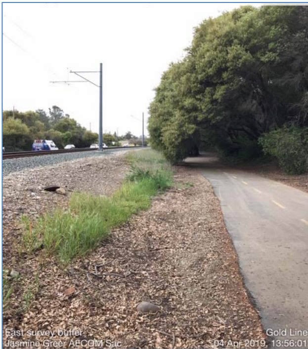
View of urban land cover: rail ballast, tracks, and bike trail, Folsom Project Segment
