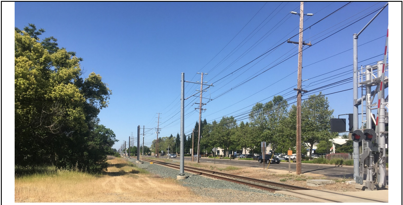
Viewpoint 5. Looking southwest along Folsom Boulevard from Aerojet Road. Railroad crossing structures, light rail track, OCS, wood power poles with overhead electrical lines, Folsom Boulevard, urban street trees, fencing, and commercial development are visible in the foreground, middleground, and background.
