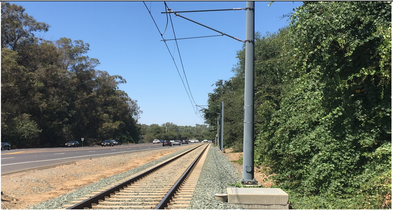
Viewpoint 3. Looking north along Folsom Boulevard from Parkshore Drive. The light rail track, gravel railroad bed, metal poles with overhead electrical lines, Folsom Boulevard, and trees in the Folsom Lake SRA and along the Folsom Parkway Rail Trail are visible in the foreground, middleground, and background.
